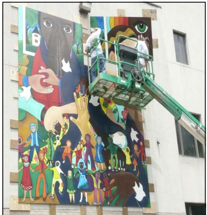
Loading the final mural panel on the wall.
